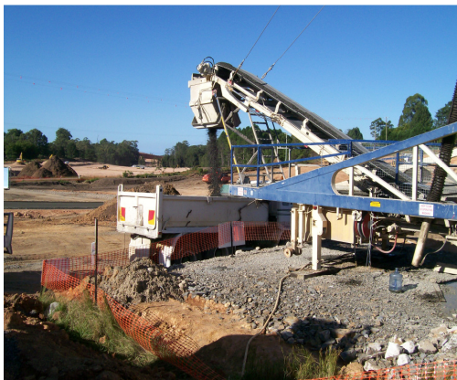
Archville Station Road – Batchplant
