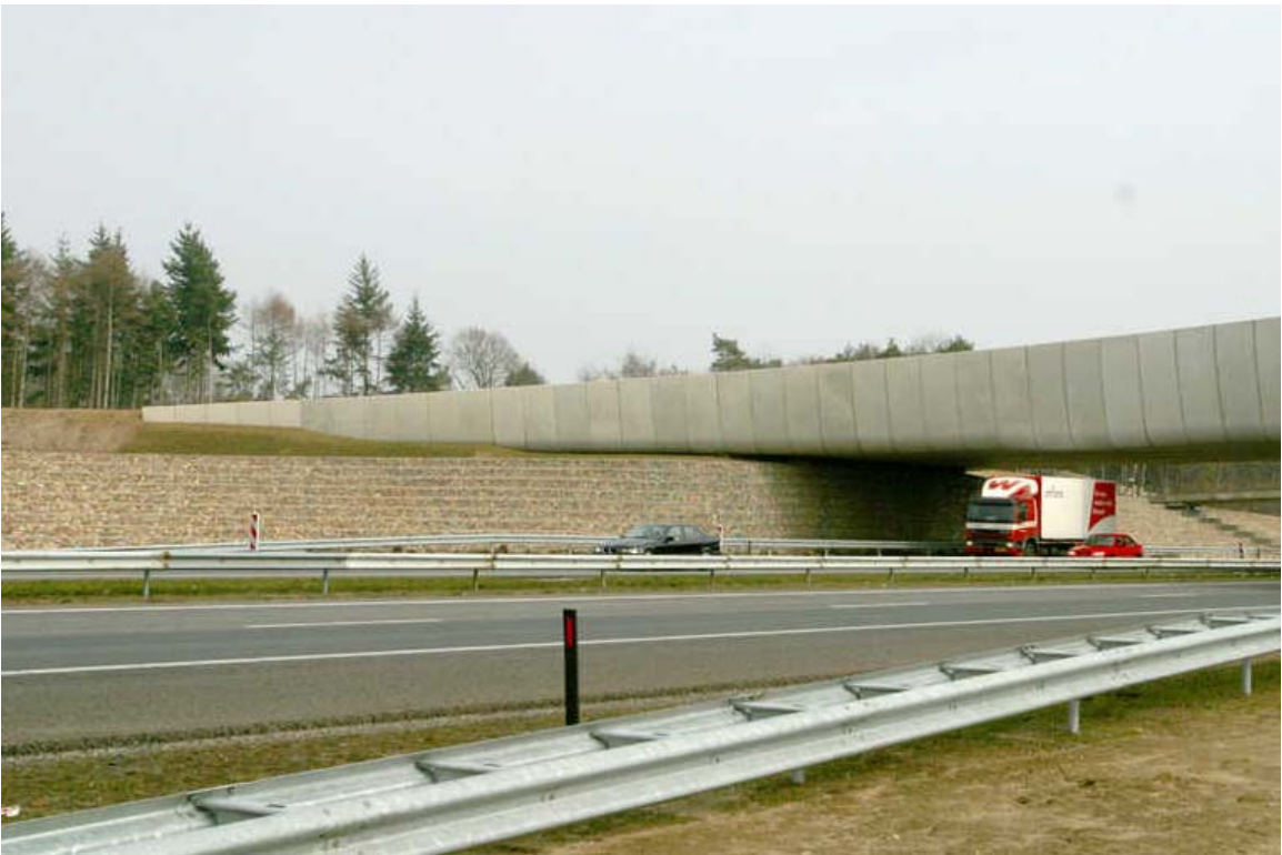
An example from the Netherlands of an overpass with solid screens.
