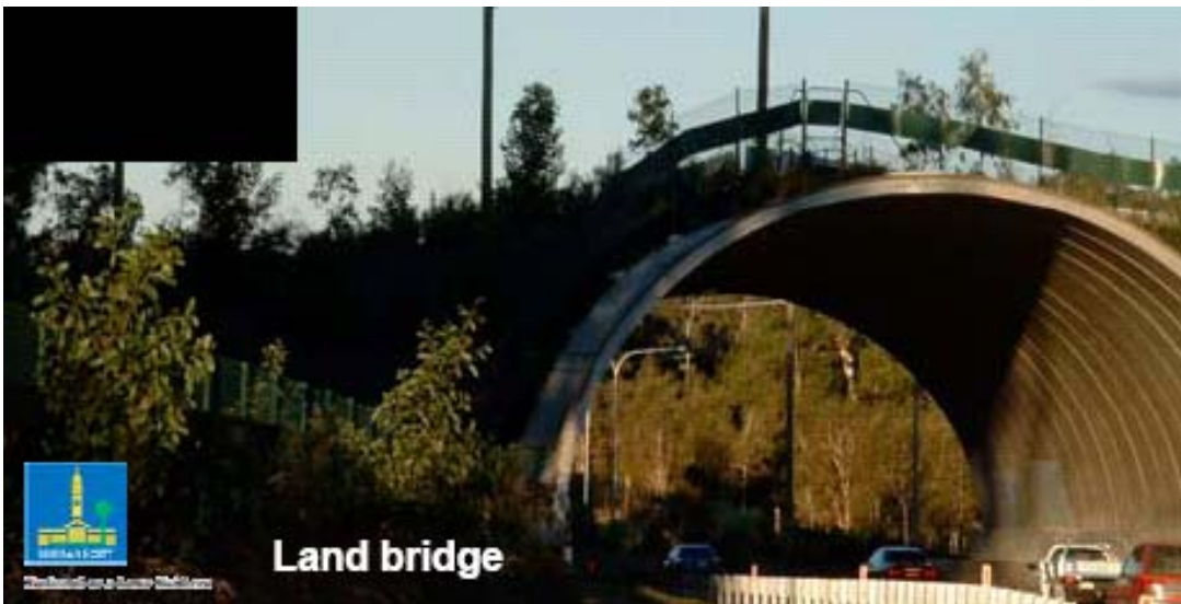
Crompton Road Land Bridge, Brisbane
